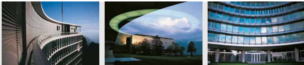
Above, left to right: West Elevation of 6th floor; View of the park from the lobby, with the light ring of the Chambord staircase reflected in the glass curtain wall; View of the lakeside facade. Opposite page, above: Peter Brabeck-Letmathe, Nestlé CEO, architects Jacques Richter and Ignacio Dahl Rocha, and David Panchaud, Nestlé Project Manager. Opposite page, below: Alpine landscape reflected in the polished marble floor of the main lobby; View of the new Oculus at the top of Tschumi's Chambord staircase.
